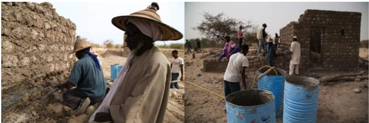
Figure 8: Reconstruction of mausoleums in Timbuktu
